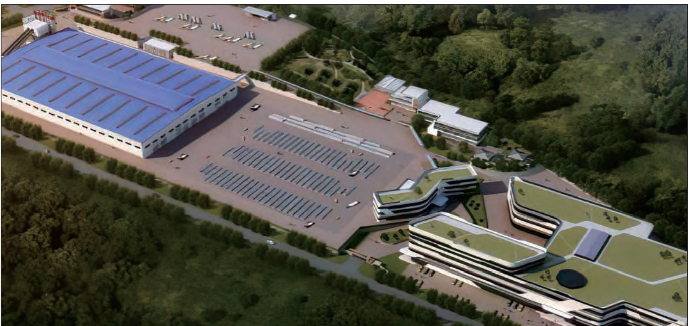
Kenya Building Industrialization Research, Development and Production Base and Construction Material Supermarket
